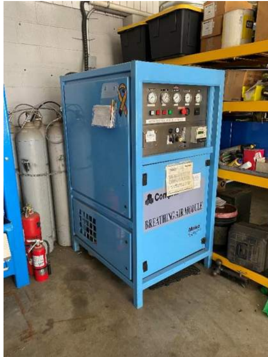
Image 9: Unanchored Equipment
