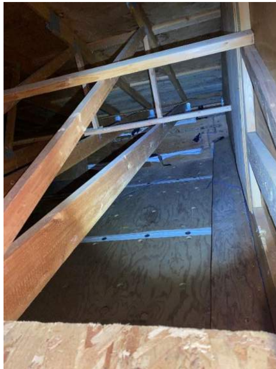
Image 8: Roof Truss Overbuild Framing
