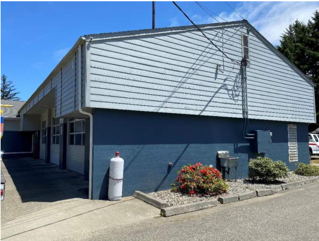
Image 4: South Elevation with URM Walls Below Wood Bearing Walls
